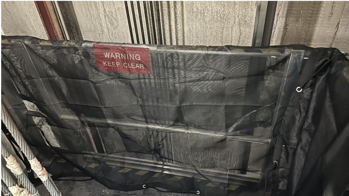
Mesh Netting hung / doubled over the guardrails.
