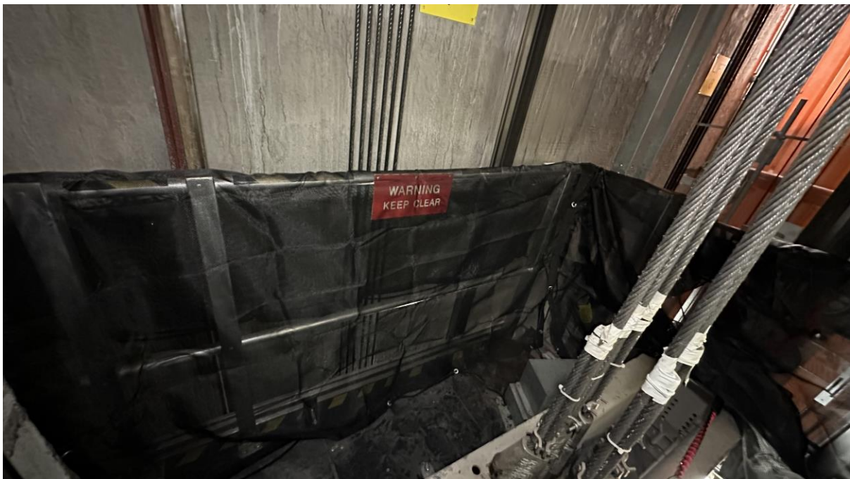
Mesh Netting hung / doubled over the guardrails.
